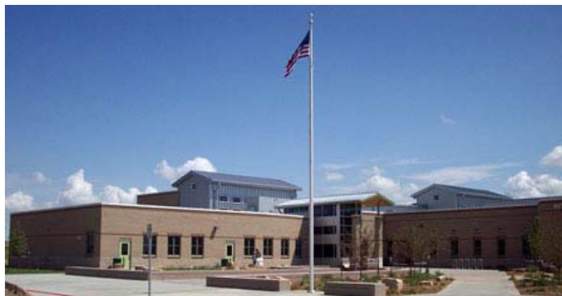
Designed by RB+B Architects, Inc., Bethke Elementary School achieved a certified rating of Three Green Globes.
